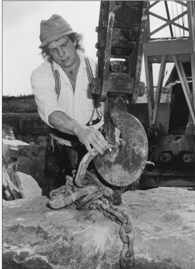
Stanley Bonfield, St Aldhelm's Quarry, 1992
